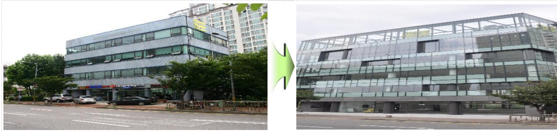
Northeast building of S tower (2011, office building)
