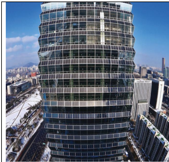
Figure 7. Solar Power Generation Facility Building
