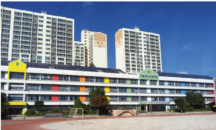
Figure 10. Case Study of Solar Light installed on a Roof
